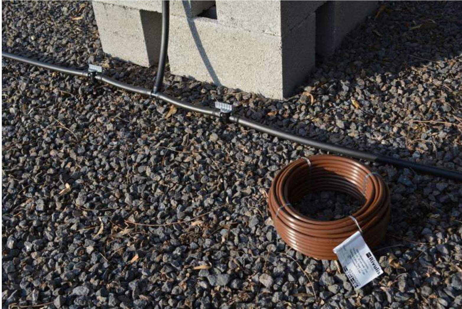
Laying the 8mm dripline along the bed, dripline length according to the design
