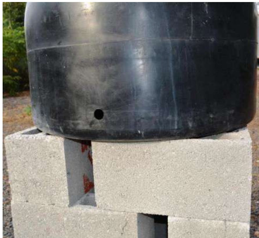
Drill hole of 25mm
