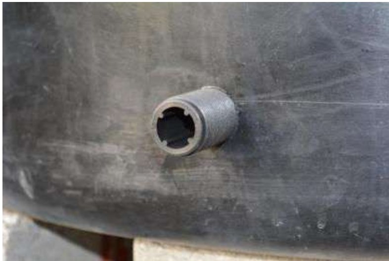
2. Insert the male threaded adaptor from the inside of the tank
