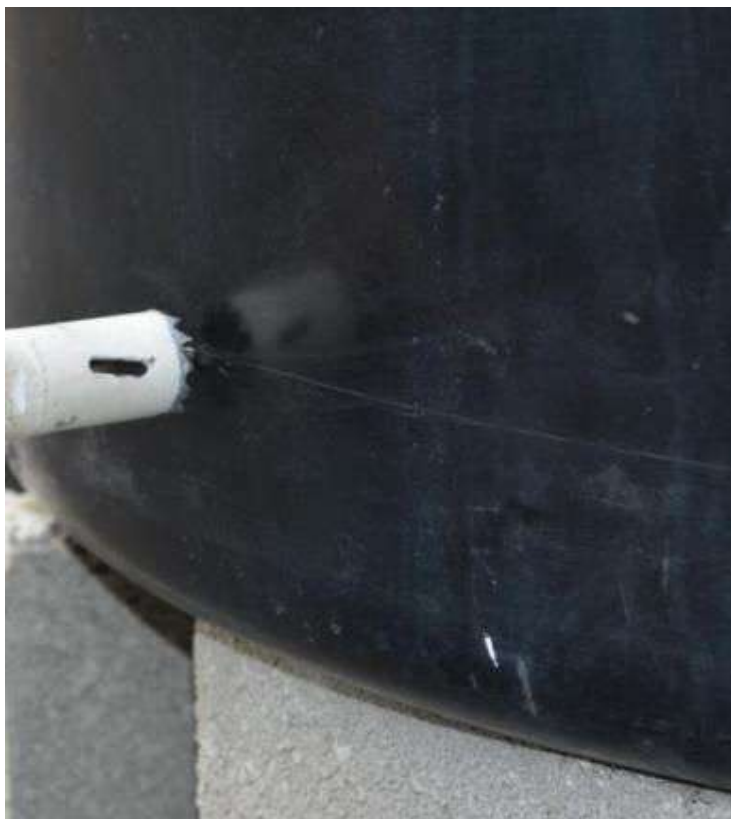
Drill hole of 25mm
